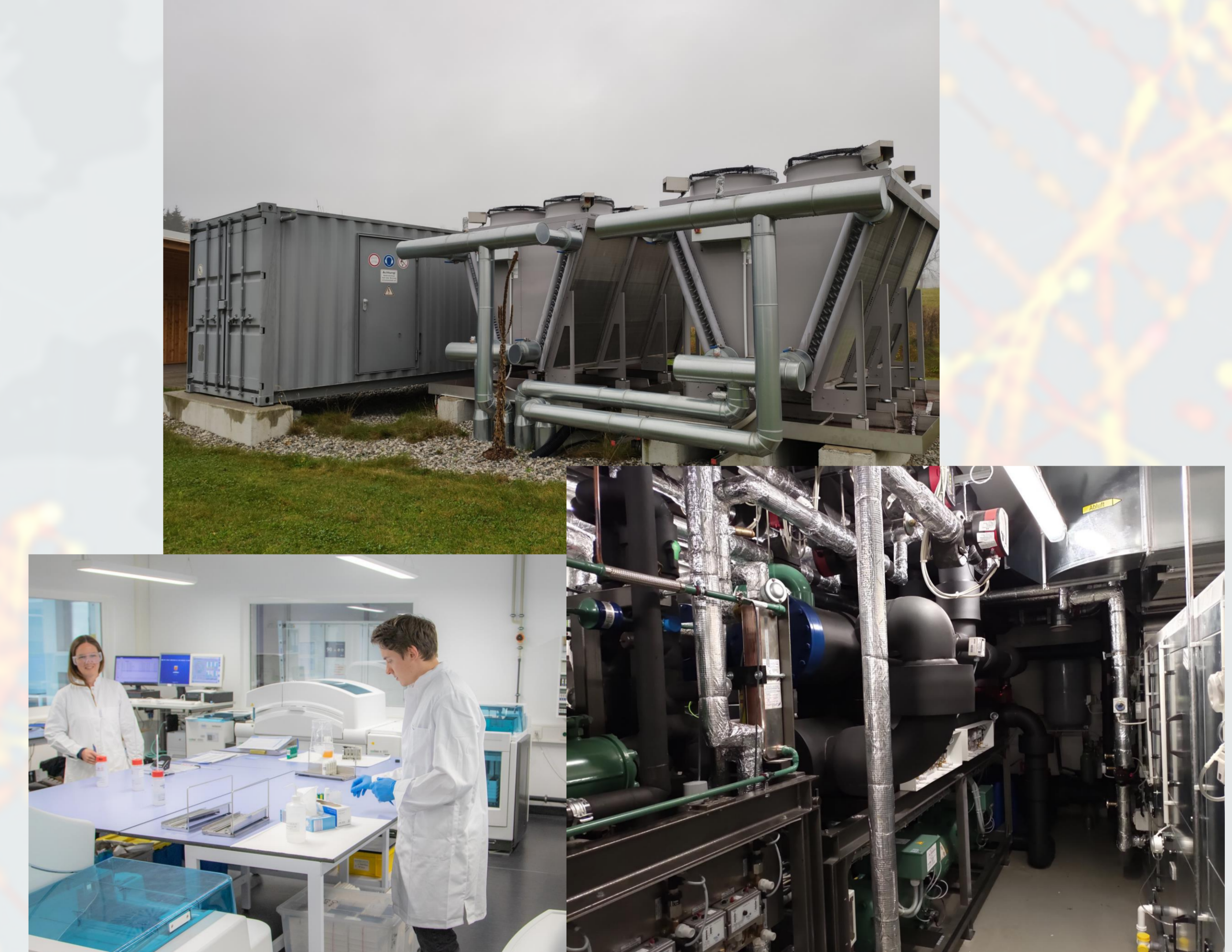
Redundant cooling engines and emergency Diesel generator at the TRIGA-S facility. Left below: High throughput Clinical Chemistry and Immunological assay Laboratory.
